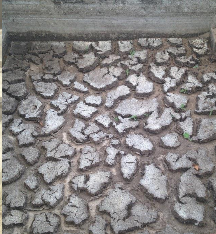
Sludge on drying bed
