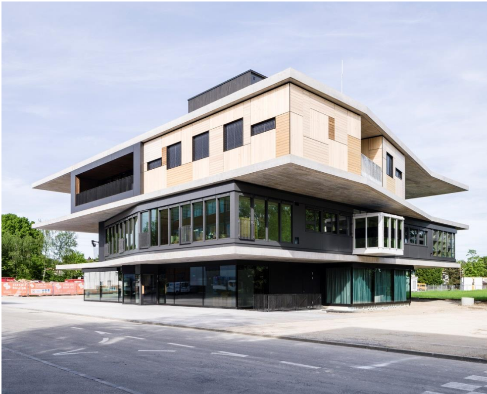
NEST building at Eawag
