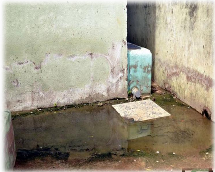
Septage overflowing
