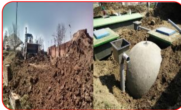
Construction of treatment plant
