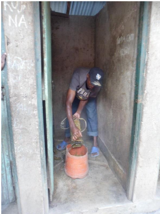
Figure 1 Manual emptier emptying a pit latrine with a bucket © GIZ/Doreen Mbalo
