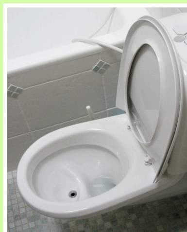
Figure 4: a Swedish flush toilet with urine diversion. Urine is typically stored in a tank for up to a year before being collected by a farmer for direct reuse as fertilizer.
