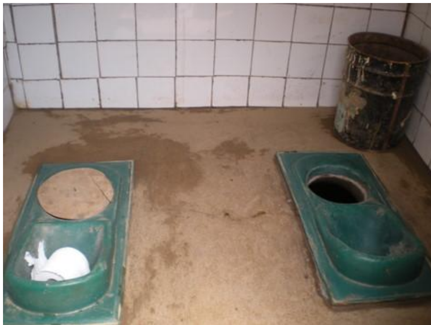
Figure 5. Urine-diverting pan of a UDDT
