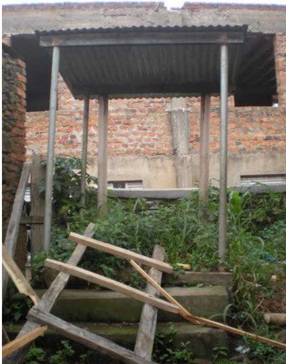
Figure 11. Partially built UDDT
