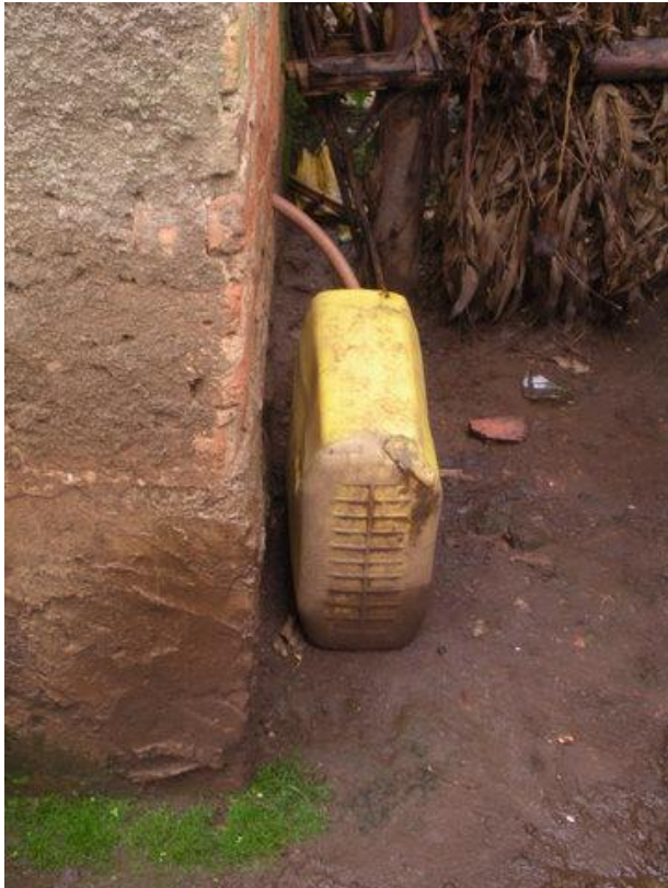
Figure 8. Tube diverting urine from UDDT into jerry can, separate from feces
