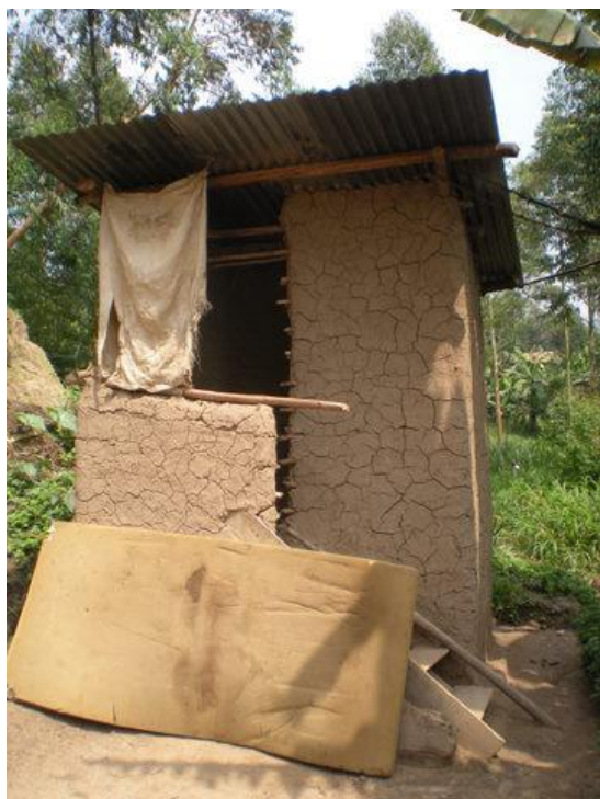
Figure 2. UDDT made from low cost materials
