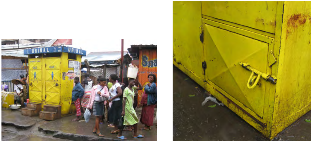
Figure 4.1: Superstructure of public urinal (left) and clack for access to storage tank (right)
