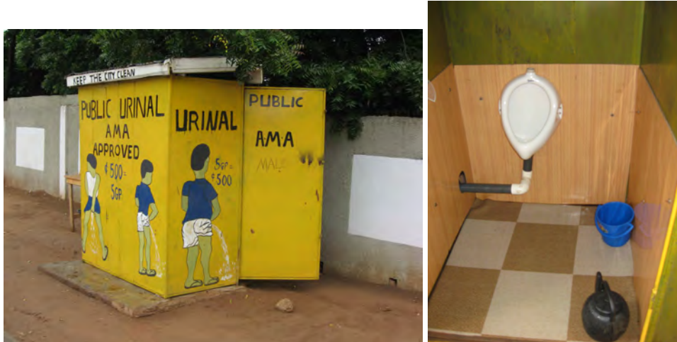
Figure 3.9: Self-constructed public urinal at Novotel Market, Accra
