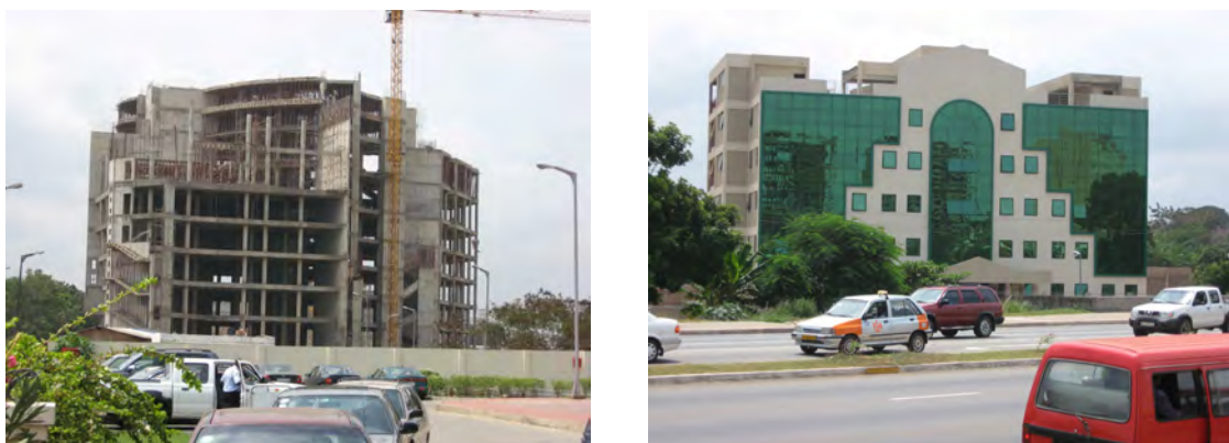
Figure 3.2: Construction site and modern office building in Accra Airport Residential Area
