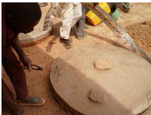
Facilitator Hamidou Kailou Constructing a round latrine slab from CREPA Niger
