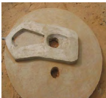
A san-plat slab does not need iron bars for reinforcement, which lowers the cost
