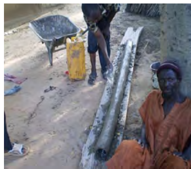
The ventpipe is made from recycled bottles, old cloth and cement
