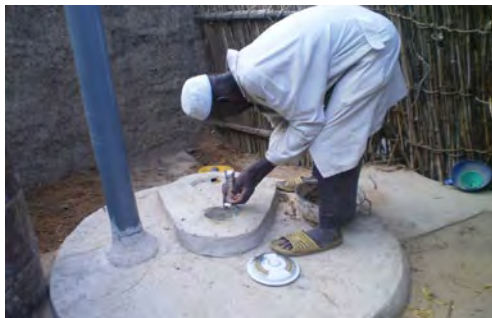
Mr Boda, facilitator in Saja Manja, verifies the pit with a flash light. The pit content should not be too humid.
