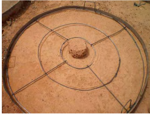
Facilitator Hamidou Kailou Constructing a round latrine slab from CREPA Niger
