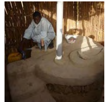
Figure 4. The dry toilet off the ground in local material except the slab and the vent pipe.
