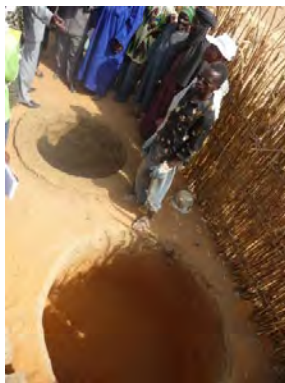
Demonstration of how the shallow composting latrines are built
