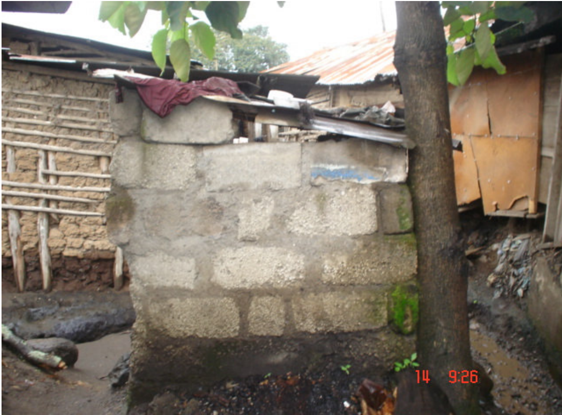
Plate 4.4: Typical Pit latrine found in residential areas of Unga Ltd
