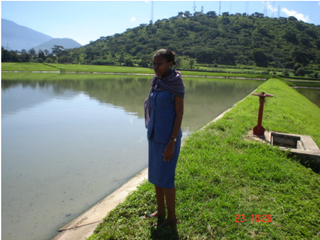
Plate 4.1:Secondary facultative stabilization pond-Lemara treatment plant.
