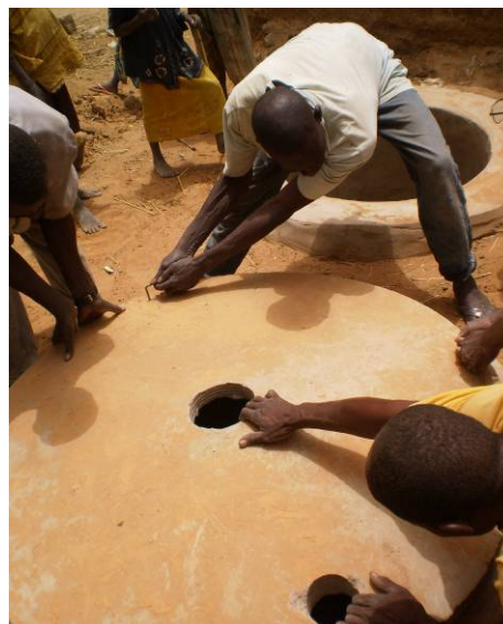
2. Place the slab on the pit.
