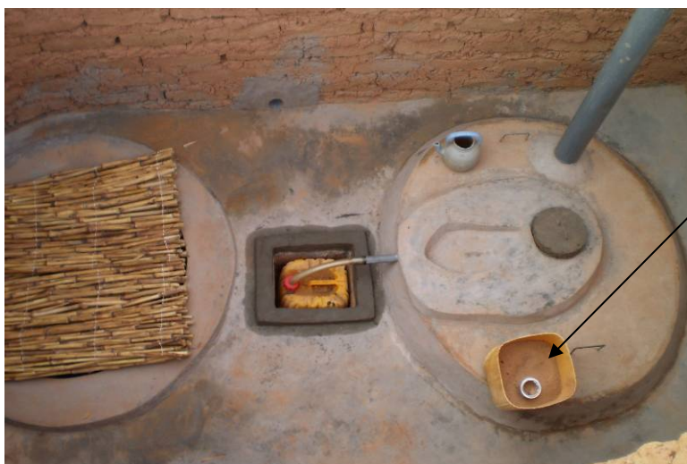
3. Cover the second pit – you can use it for composting while waiting for the first one to fill up.
