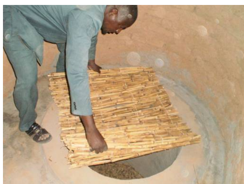
3. Cover the second pit – you can use it for composting while waiting for the first one to fill up.
