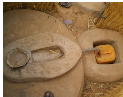
Urine from a composting toilet.
