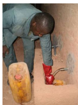
5. Replace the pipe with the lid on the new jerry can.
