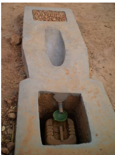
An improved urinal can be made in cement, on the behalf of the household.
