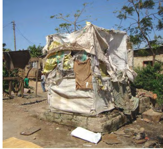
Picture 7: Standard. raised pit latrine
