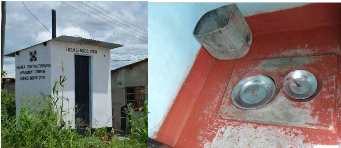
Picture 15+16: Urine-Diversion Dry Toilet of NECOS, exterior and interior
