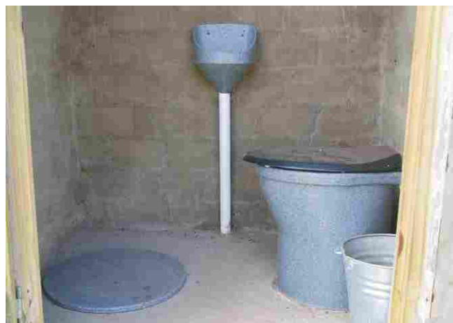
The inside of a UD toilet
