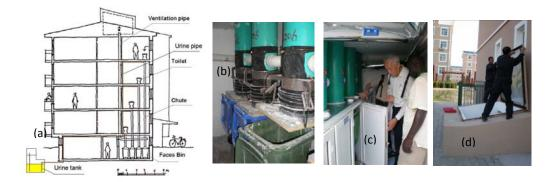
**Figures 3-6a to 3-6d.** The EETP faecal collection system. (a) The layout of UDD toilets, faecal chutes, and bins in the basement. (b) The movable bin covers attached to the faecal chutes. (c) The sealed cabinets housing the bins. (d). The covered pit access to the basements. [(a) from Zhu, 2008 and (b-d) A. Flores, taken in August 2007.]
