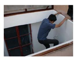
*Figures 4-4a and 4b.* Views of the covered pit access to the basements at the EETP. Bins are moved in and out of the basements using a hoist attached to the bin collection truck. [A. Flores, taken 5 September 2007.]
