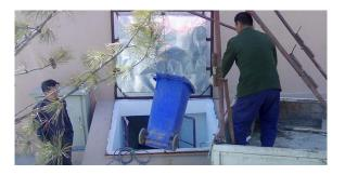
*Figure 7-11.* Collection of faecal bins from the basement. [Source: http://www.adb.org/, accessed 11 November 2009.]
