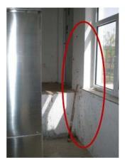
*Figure 7-13.* Contamination of the composting facility walls with faecal material from the bins. The sifter is on the left. [A. Flores, taken 24 April 2009.]
