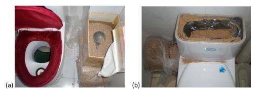
**Figures 4-3a and 3b.** Sawdust use in the UDD toilets. (a) Example of a well-maintained UDD toilet with a sliding plate mechanism. Note that the household is using a box instead of the dispenser. (b) Example of the mess that can be caused by sawdust. [A. Flores, taken September 2007.]
