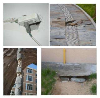
Figures 7-16a to 16d. Examples of poor construction at the EETP. Clockwise from top left: badlyinstalled electrical socket, poorly done paving and building foundation, and disintegrating concrete decorations in the outdoor play area. (Source: USTB-CSES and Envirosystem Ltd., 2008)
