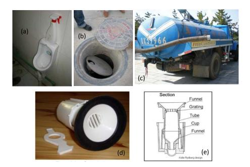
**Figures 3-5a to 3-5e**. The urinal and urine collection system at EETP. (a) The urinal with an Strap. (b) Access to a urine storage tank. (c) The vacuum truck that collects and transports urine. (d) The paraffin-oil odour trap. The key on the left is to be used for disassembling the trap for cleaning. (e) A cross-section drawing of the odour trap. [(a-c) A. Flores, taken in September 2007 and (d-e) from Zhu, 2008.]
