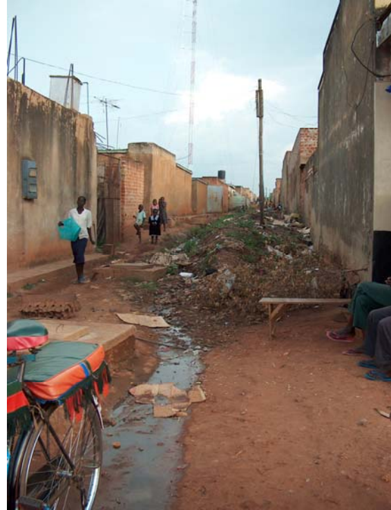
Picture 1: Wastewater discharged from houses onto road (Gulu, Northern Uganda)
