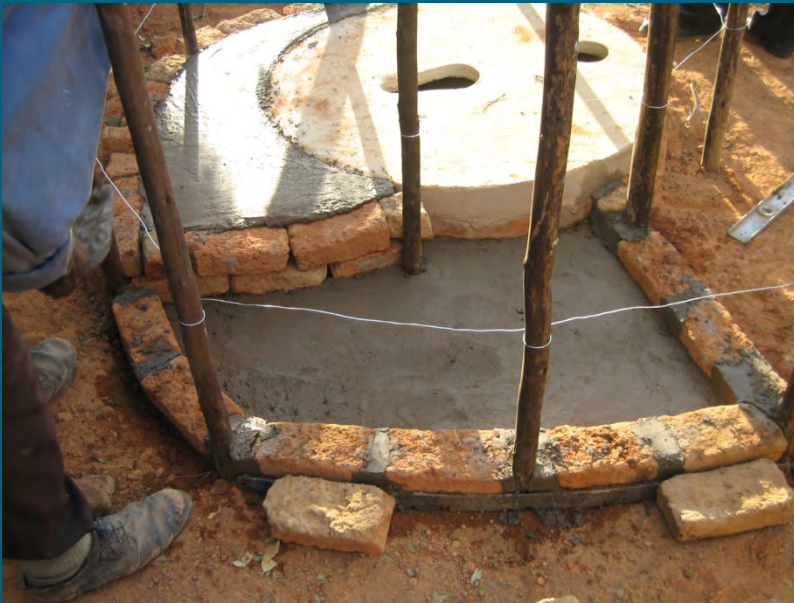
Slab extensions made for spiral structure (grass and brick)
