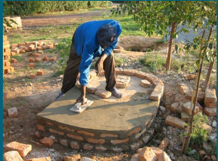
Slab extensions made for spiral structure (grass and brick)
