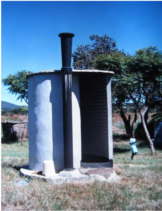
On the left a classic Blair Latrine built at Henderson Research Station in 1976. On the right the same unit is still in use on the wide pit (1.5m) in 2006.
