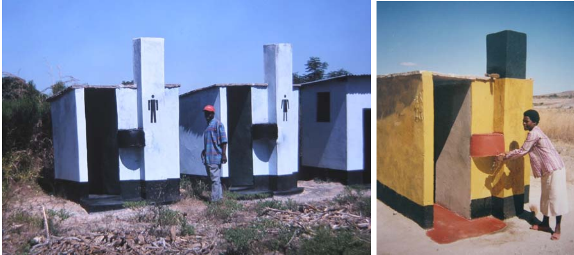
The most commonly built model was a brick built square spiral built without a door. The vent was also made of brick. Later brick built Blair Latrines were often fitted with hand washing facilities.
