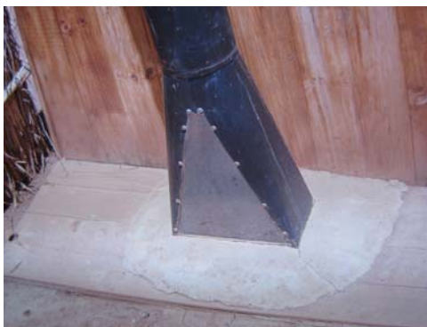
Experimental vent pipe with fly trapping window. Fly trap with flies.
