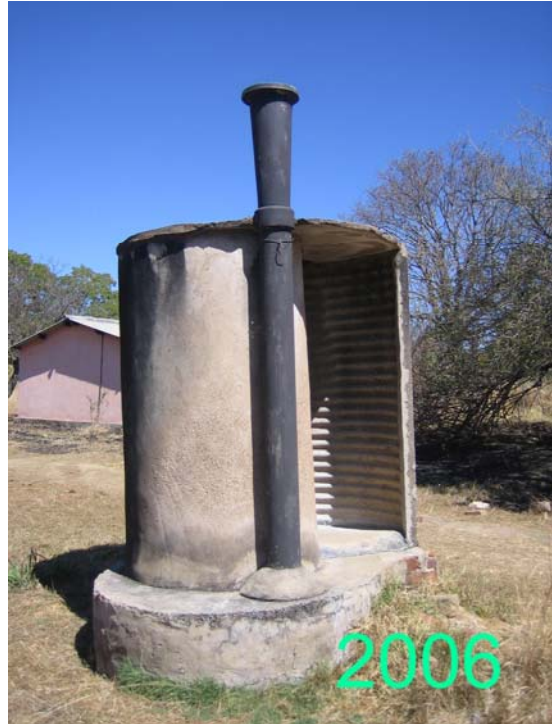
On the left a classic Blair Latrine built at Henderson Research Station in 1976. On the right the same unit is still in use on the wide pit (1.5m) in 2006.
