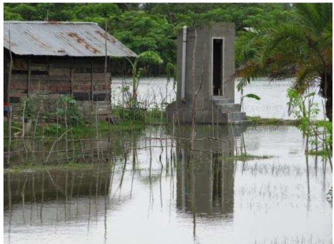
Fig. 13: UDDT (on the right) prevents excreta contamination during cyclone Aila, May 2009, which hit the area shortly after construction of UDDTs was completed (source: Laxman Kharal Chetty, 2009).
