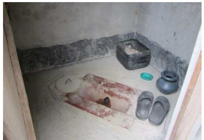
Fig. 11: After approximately two years in use, the squatting pan and toilet on the whole was being well maintained (source: Shahid Kamal, May 2011).
