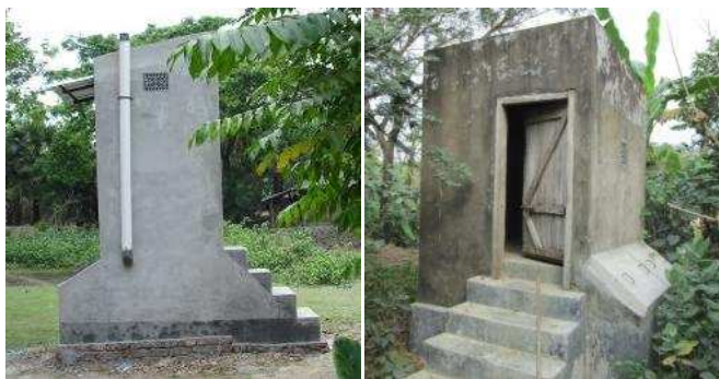
Fig. 5: The two UDDT designs used, on the left the faecal vaults are at the rear and on the right they are on the side of the superstructure (source: Antoine Delepière, 2009 (left) and Shahid Kamal, May 2011(right)) 5 .
