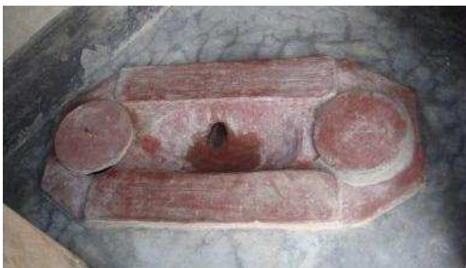
Fig. 8: Installed squatting pan (source: Laxman Kharal Chetty, 2009).
