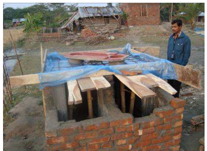
Fig. 4: Vault and slab construction (source: Antoine Delepière, 2009)
