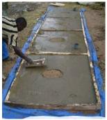
Photograph 10 Casting Fossa alterna slabs
