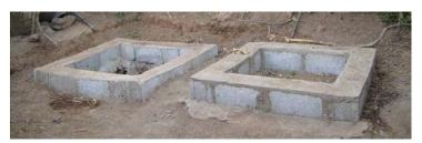
Photograph 9 Fossa alterna ring beams
