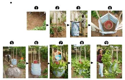
Figure 3 Steps followed to construct a Greywater tower
