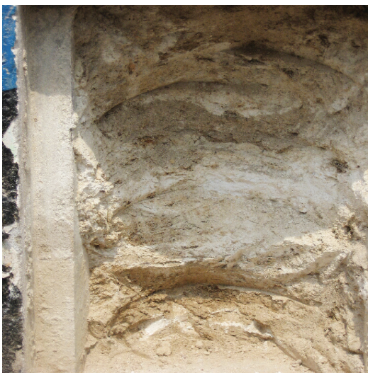
Photo 19: Layers of safe material in the chamber
