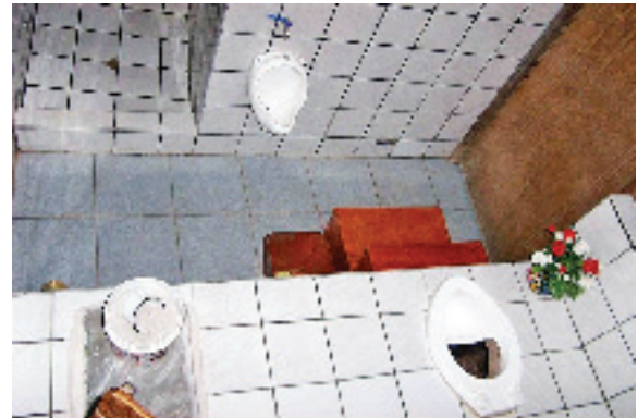
Foto 8: Two chamber UDDT with recessed eco-toilet
