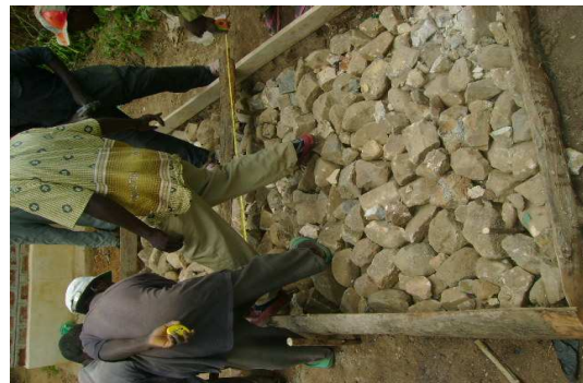
Laying the foundation for UDDT and rain water harvesting Ferro-cement Tank
