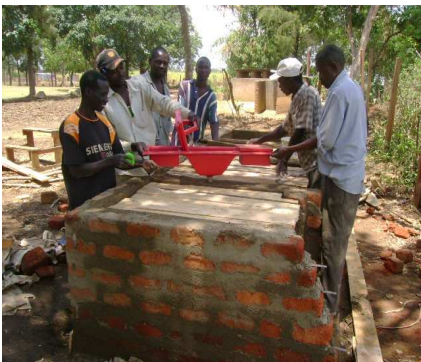
Fixing of the squat pan before casting of slab in UDDT
