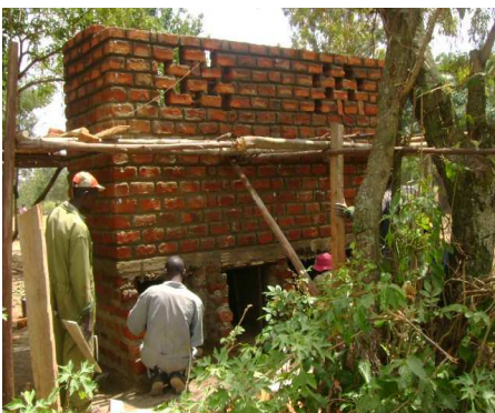
Wall construction for the UDDT by the technicians with brick vent openings
