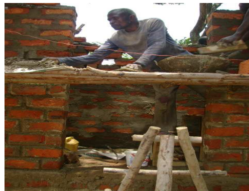
Wall construction for the UDDT by the technicians with brick vent openings
