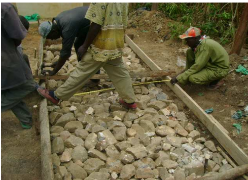
Laying the foundation for UDDT and rain water harvesting Ferro-cement Tank
