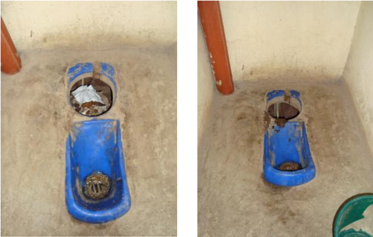
Figure 12: Signs of cross-contamination (source: L.Kraft, May 2011)
