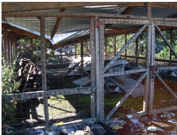
Figure 19: Left: MEWAREMA drying shed which was destroyed by strong winds Right: Donkey cart for transport of faeces (source: L.Kraft, May 2011)
