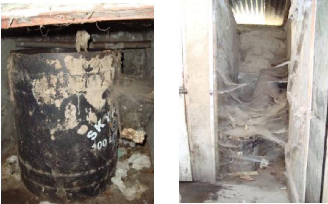
Figure 17: Left: Container for faeces collection (in use) Right: Old, filled up faeces container stored in the bathroom (source: L.Kraft, May 2011)
