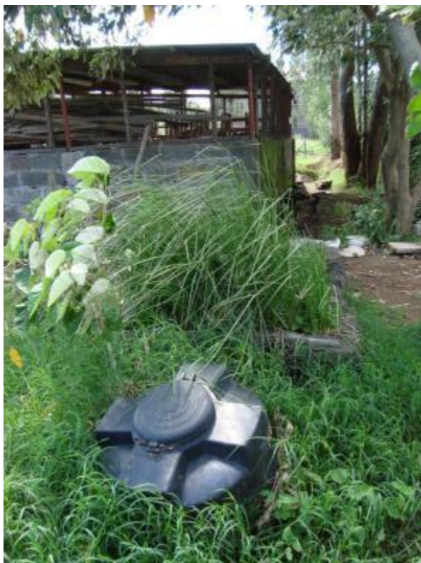
Figure 15: Left: Greywater treatment system with settlement tank Right: Outlet of treatment system with very little outflow (source: L.Kraft, May 2011)
