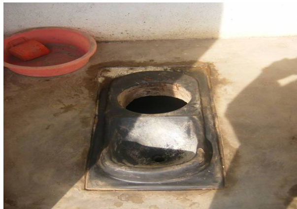
Figure 4-5: inside the room of UDD toilet at Nyamagabe secondary school
