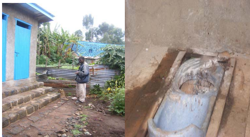
Figure 4-9: Public UDD toilet in Rugarama business centre
