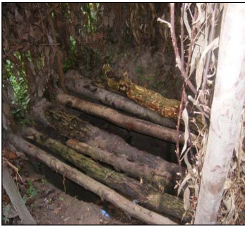
Figure 4-6: Pit latrine in Gahunga village
