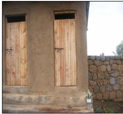
Figure 4-7: UDD toilet for household in Gahunga
