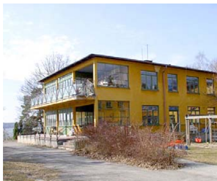
Figure 1: Gebers Building (source: VERNA Ecology Inc.)
