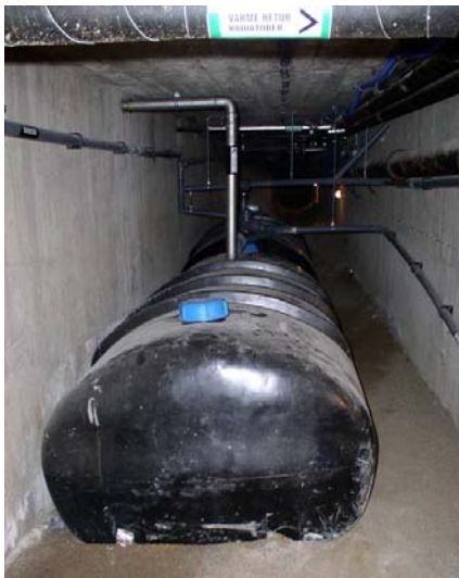
Figure 4: Urine Collection Tank (source: VERNA Ecol.)
