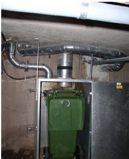
Figure 5: Faeces Collection Bin (source: VERNA Ecol. Inc.)
