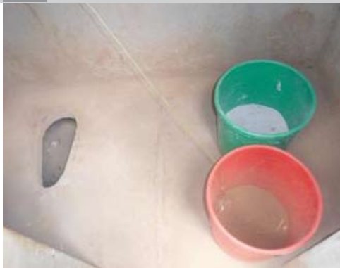
→ Inside the clean girls' fossa alterna toilet
