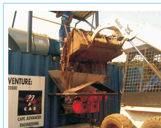
Figure 37 a,b: Semi-dried sludge being loaded into the machine
