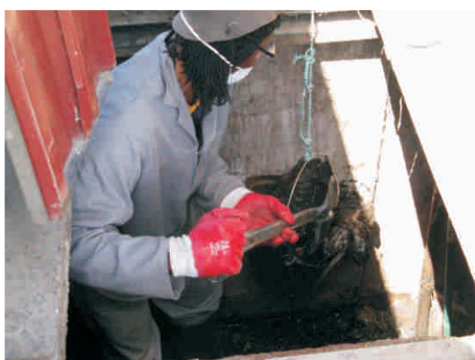
Figure 23 : Manual emptying of chambers
