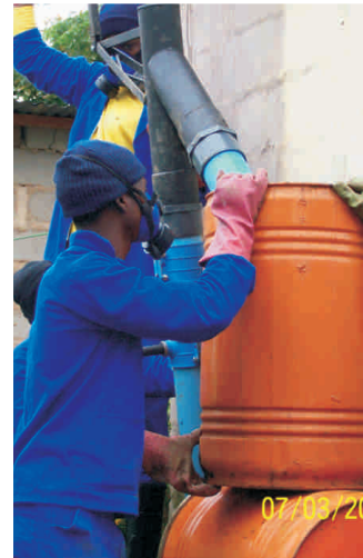
Figure 33: Using specialised tools to extract wet sludge from septic tanks
