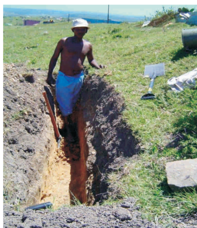
Figure 24 : On-site deep burial of sludge
