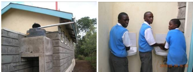
Figure 14 Roof water harvesting system and students washing their hands after visiting toilet (Source: Muchiri, 2009)
