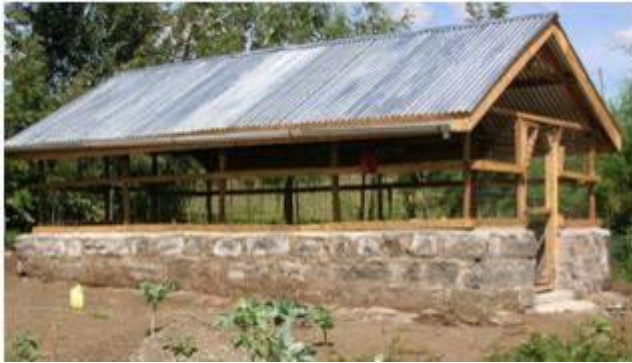
Figure 13 Drying shed for processing faecal matter from the UDD toilets (area 6 m x 3.6 m) (Source: Muchiri, 2009)
