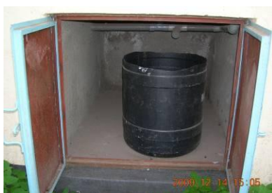
Figure 10 Interior of a faeces collection vault with a 50 litre container to collect the faeces (Source: Muchiri, 2009)
