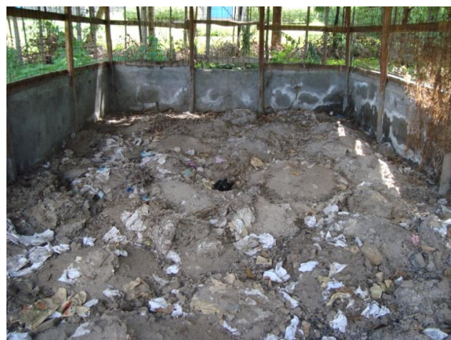
Figure 17 Dried faeces mixed with not degradable materials inside the drying shed (Source: L.Kraft, May 2011)
