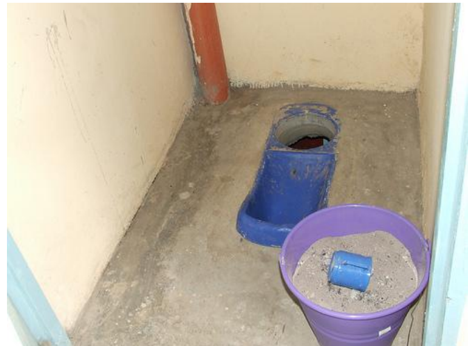
Figure 7 Inside of the UDDT, showing urine diversion squatting pan and bucket of ash (Source: Muchiri, 2009)
