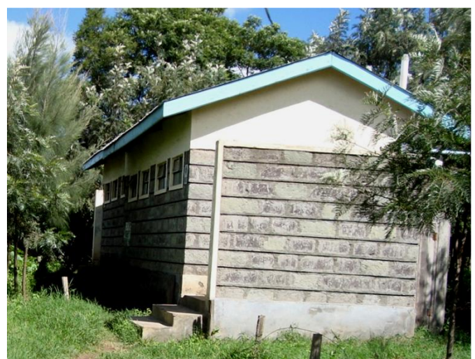
Figure 3 The UDDT facility at Crater View Secondary School two years after construction (Source: L.Kraft, May 2011)
