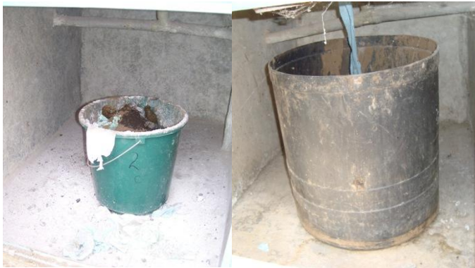
Figure 10 On the right 20 liter container in a single vault (2009). Left: 70 liter container used during the field visit in 2011 (L.Kraft, May 2011)
