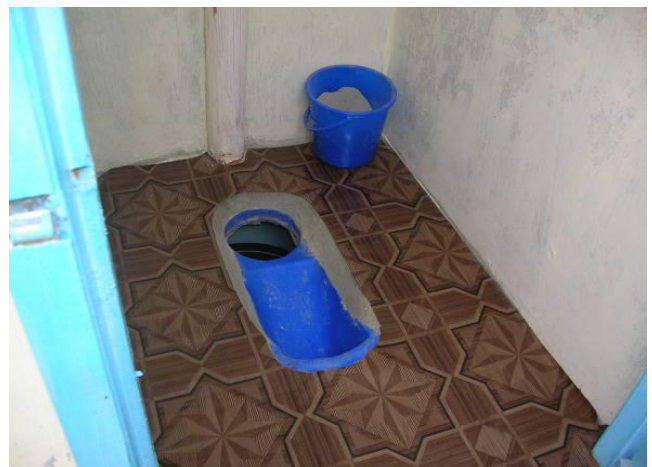
Figure 6 Inside the single vault toilet at the church showing the urine diversion pedestal and a container of ash.
