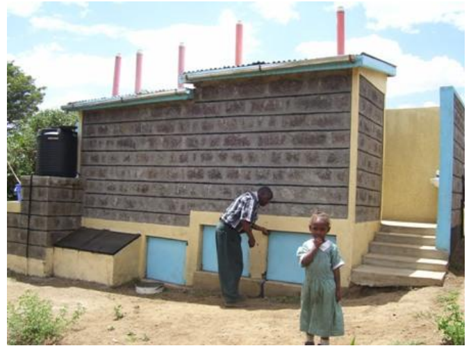
Figure 11 The rear of the UDDT showing the single vaults and the solar drier for the double vault
