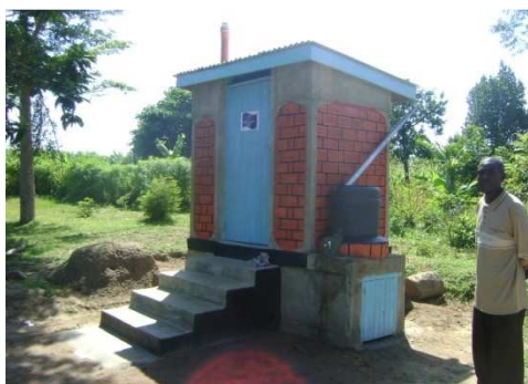
Photograph 1. Household double vault UDDT with rain water harvesting and hand washing facility to the right.
