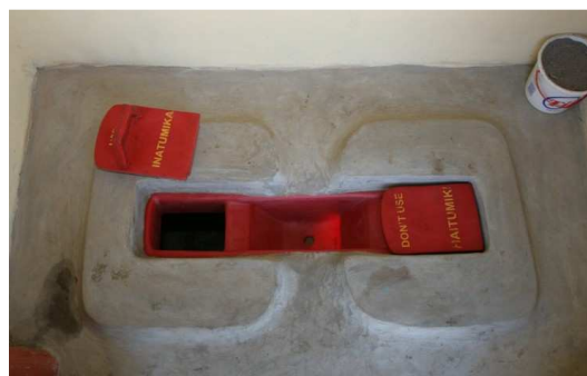
Photograph 2. Inside of household double vault UDDT with urine diversion squatting pan (with two faeces outlets) and ash bucket.
