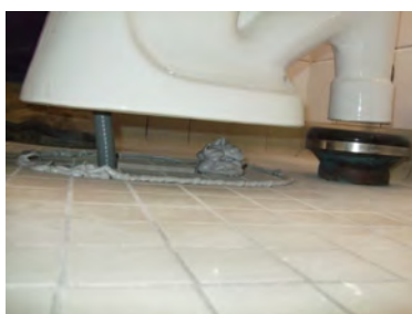
Urine pipe installed through the floor
