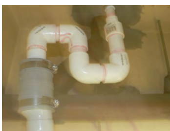
Water trap constructed under floor
