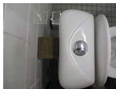
Toilet retrofit showing space from back wall
