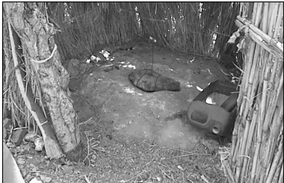
Stone Slabs on Arborloo – SNNPR, Ethiopia Alemayehu WIMariam for CRS.
