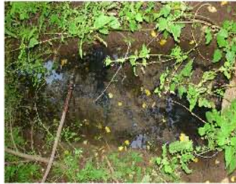
Fig. 2: Illegal pipe connections of several houses, which wastewater is discharged into the park.
