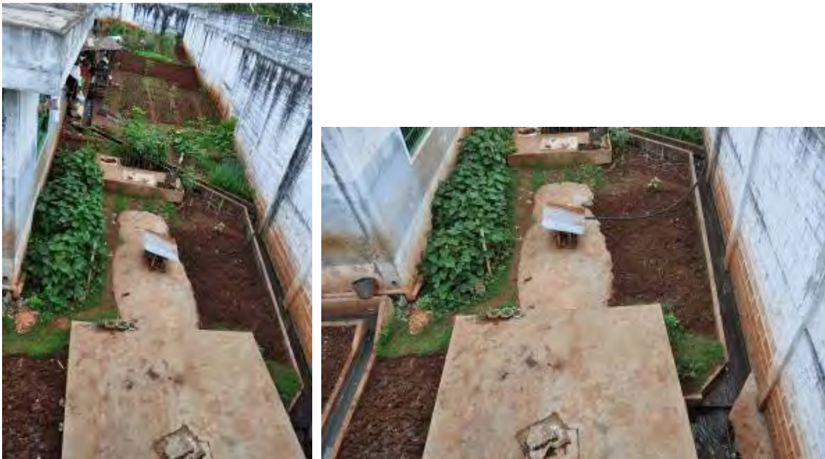
Figure 4. Photos of the biogas reactor, inlet canals of wastewater, and the outlet biogas pipe
