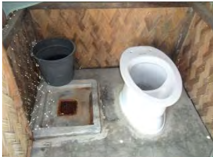
Figure 2. An Ecosan UDDT installed in Barangay Parian Oeste (left) and a view inside the unit (right), showing the UDDT bowl, the anal washing drain, and a water bucket for anal washing. The ash bucket is also present, but out of view of the photo.
