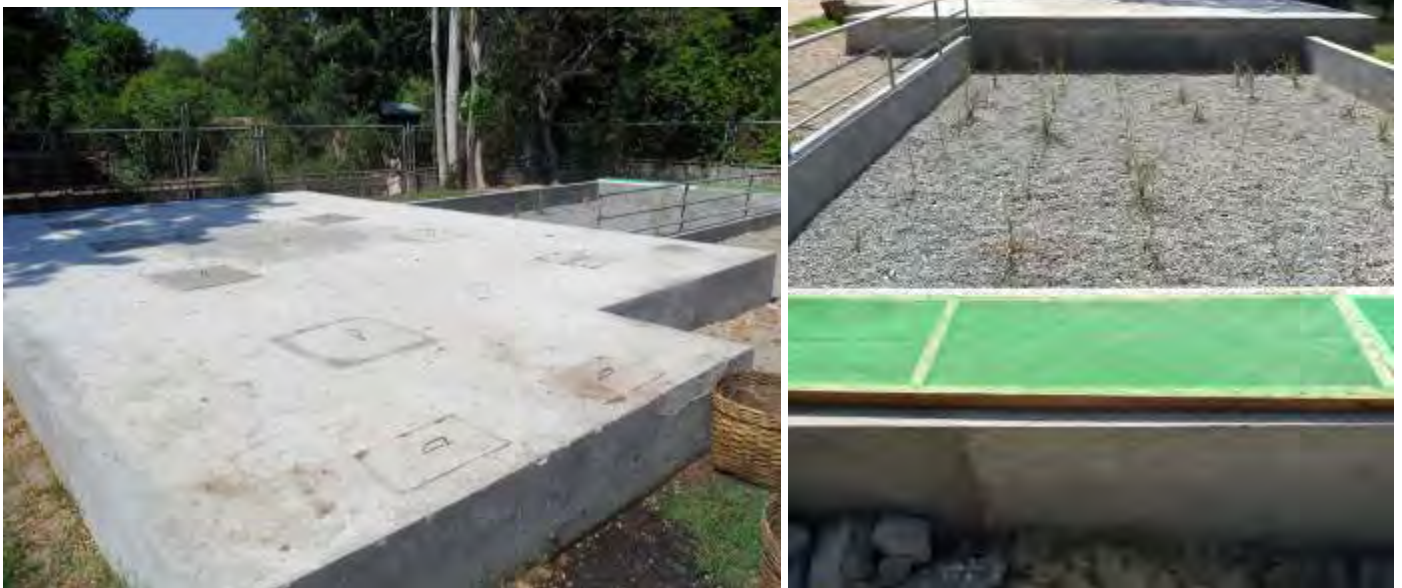
Figure 2. Photo of the ABR/AF, HGF, and indicator pond (under the green mesh) units of the DEWATS
