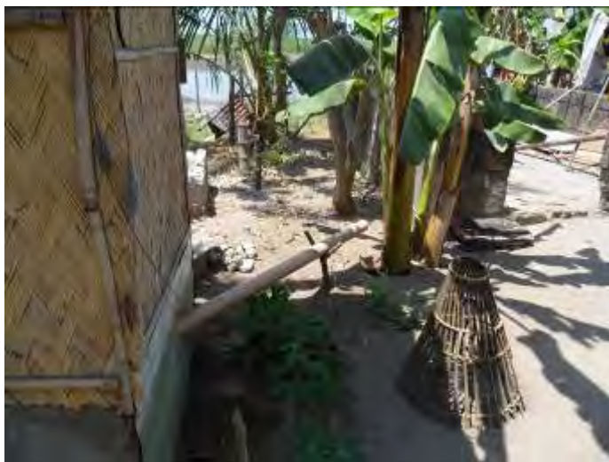
Figure 3. The floor drain pipe for anal wash water draining to an adjacent tree (left), and the ground level of the urine and feces containers underneath the UDDT superstructure (right)
