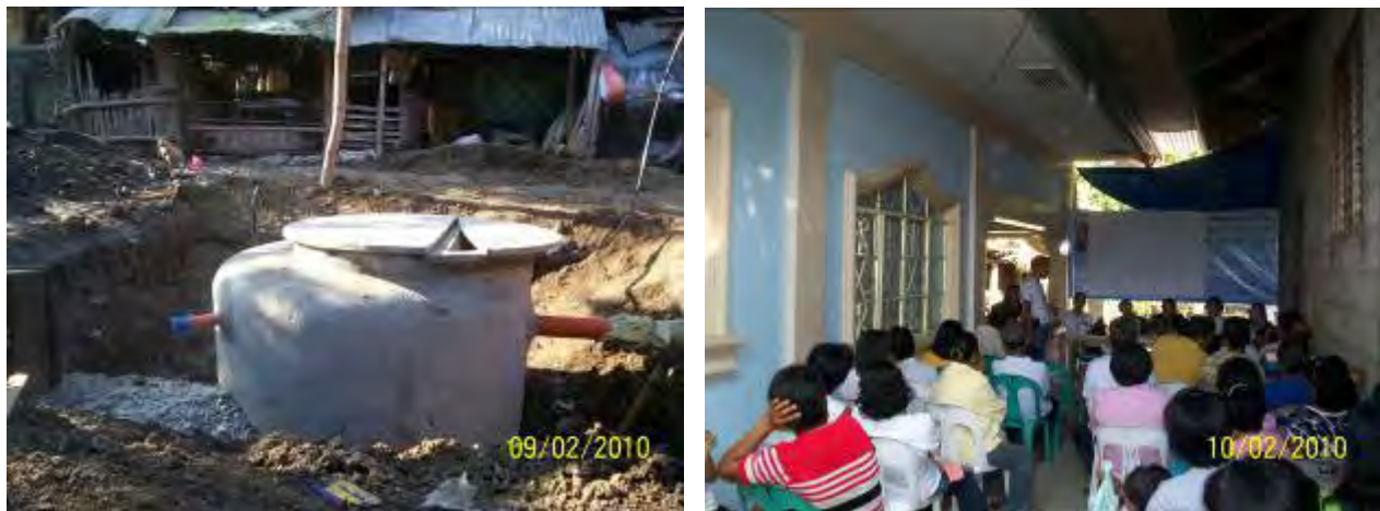
Figure 3. A photo of a nearly complete biogas reactor (left) and of one of the IEC sessions (right)
