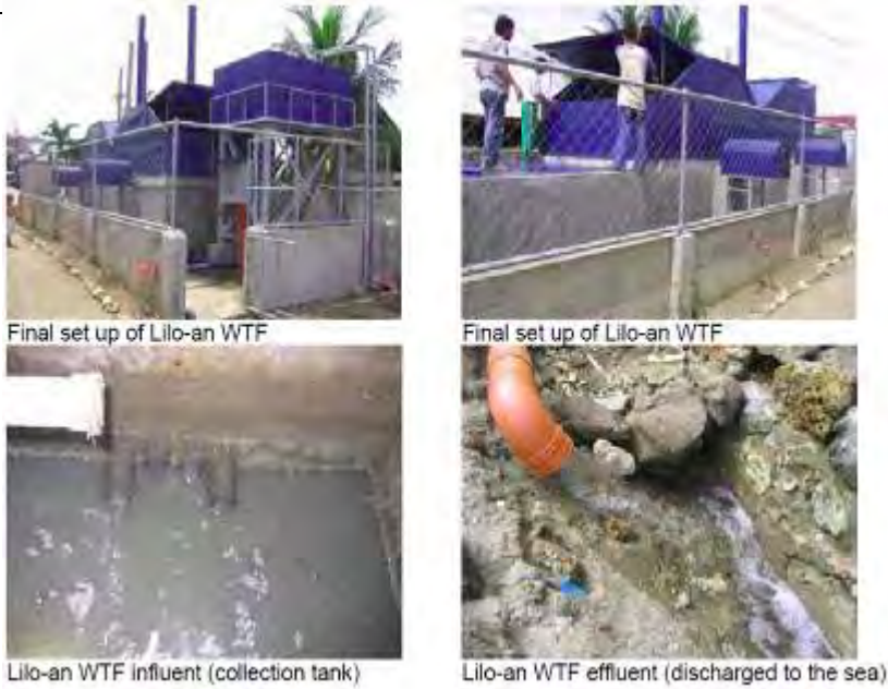
Figure 4: The completed WTF and images of the influent and effluent quality
