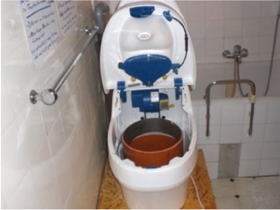
Collection and treatment chamber
