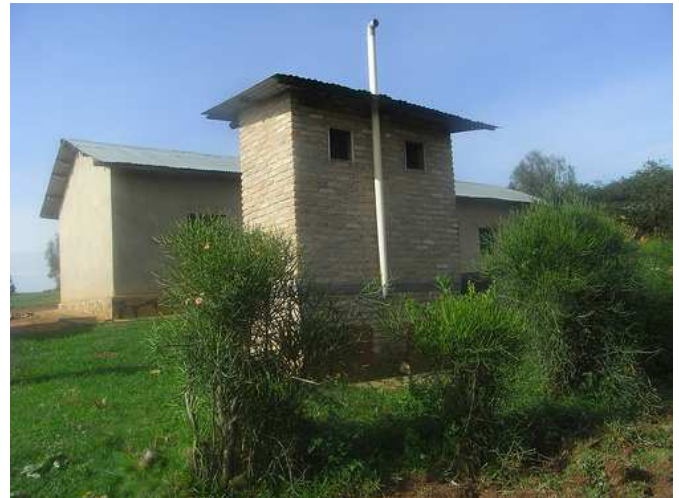
Fig. 7: Back view of the two UDDTs for teachers in Kiruhura primary school. At the base (covered by the bushes) are the access doors for the faeces vaults.
