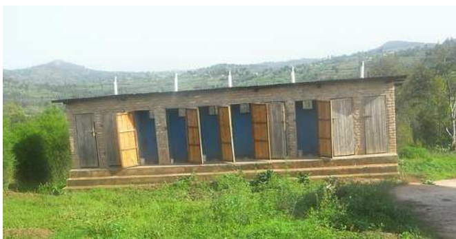
Fig. 5: Toilet block with 10 single vault UDDTs at Kiruhura Primary School (teachers have another 2 UDDTs built separately). Five cubicles are for boys, five for girls 8 .
