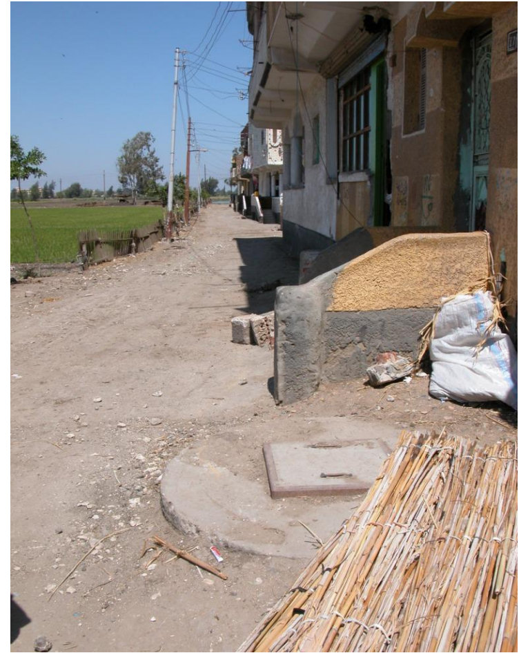
After implementation of the sewage system
