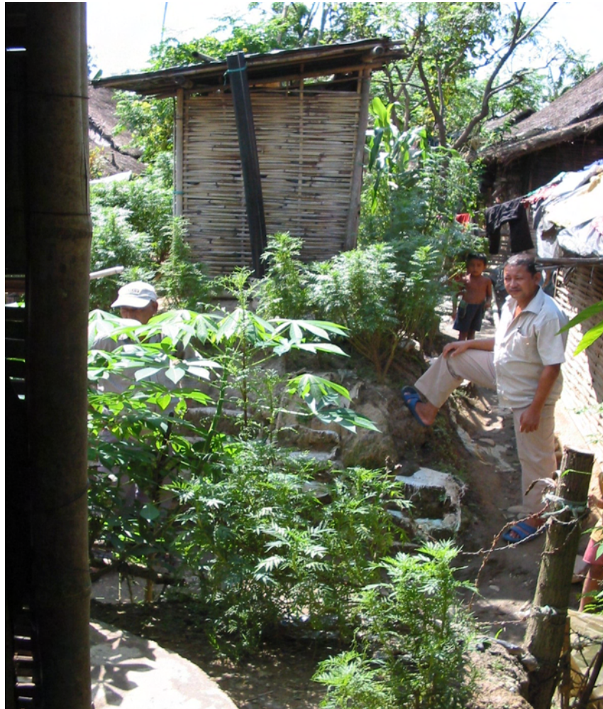
Photograph.2 Raised VIP latrine in low land area of Sanischare Bhutanese refugee camp
