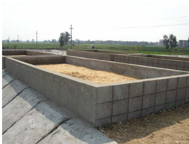
Figure 4. Sludge drying beds at El Mofty El Kobra
