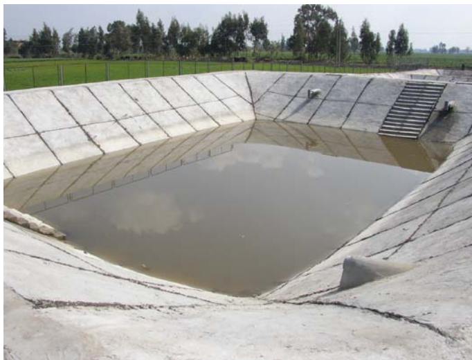
Figure 3. Anaerobic pond at El Mofty El Kobra
