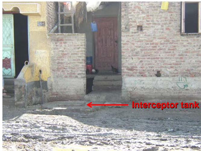
Figure 1. Interceptor tank serving a single household at El Mofty El Kobra
