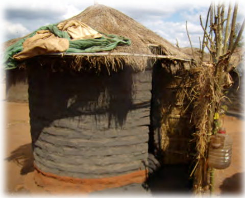
Figure 4-5: Pit latrine (with hand washing facility) in Msenda, Lilongwe district
