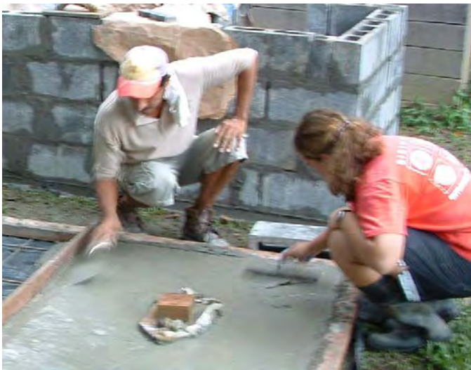
Figure 15. Smoothing out concrete with flat mason's trowel
