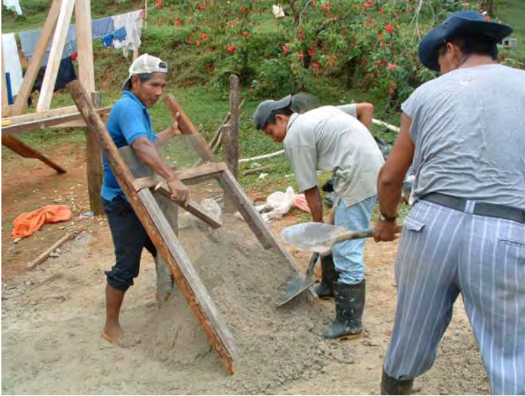
Figure 11. Sifting sand to use for mortar.
