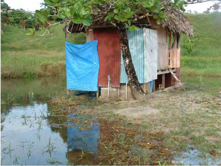
Figure 1. The author's compost latrine (and house) surrounded by water, after a high tide and heavy rainfall caused the nearby stream to swell. Note – Contents remained dry
