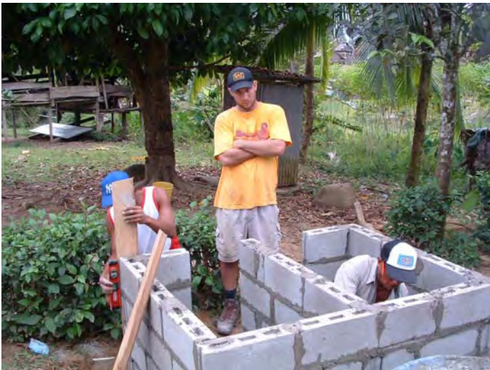
Figure 17. Erected Walls With 2-5 cm Filled-in Gaps Between Blocks
