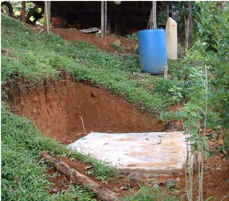
Figure 13. Leveled hillside with concrete floor of latrine showing
