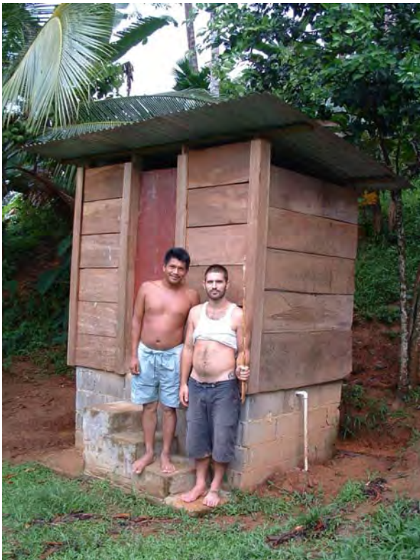
Figure 9. Typical compost latrine in the Bocas del Toro area of Panama. Note – PVC tubes (emerging from wall) transport urine from the seat to a soak pit next to latrine.
