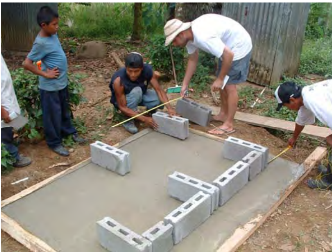
Figure 16 – Aligning concrete blocks before placing with mortar.
