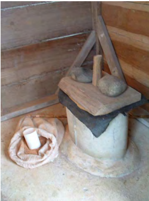
Figure 26. Example of a tight fitting cover for a latrine seat, using wood and heavy stones. Note the bag of sawdust (left of seat) that is used as a soak material.
