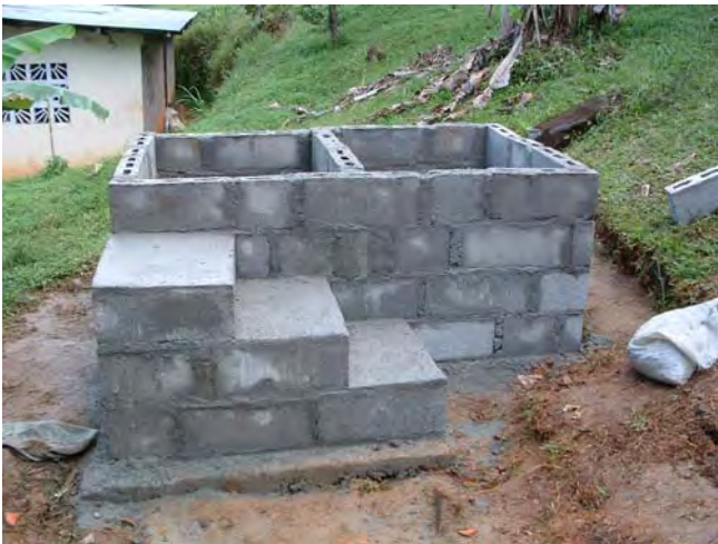
Figure 20. Staircase for compost latrine made from concrete block.
