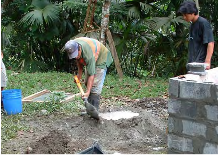
Figure 12. The “volcano” style of mixing of concrete
