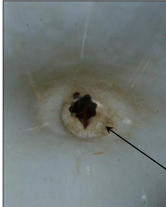
PHOTO BAD T4b: Early SOIL UD toilet seat, drainage holes forceably enlarged to unblock drainpipe.
