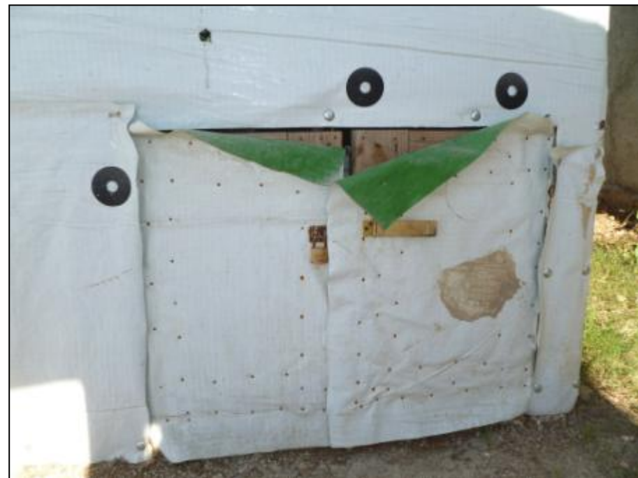
PHOTO T12: Close-up on chamber doors
