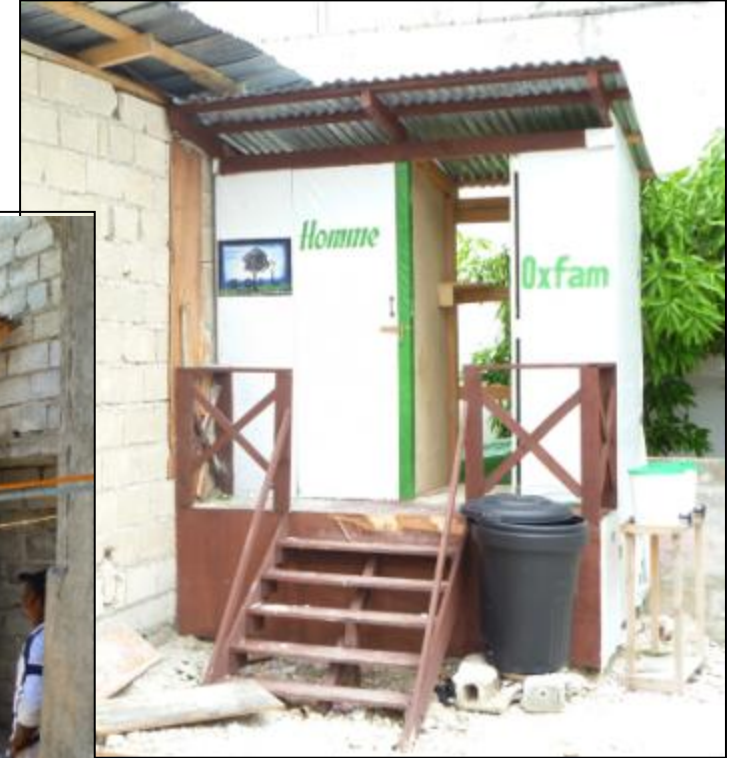
PHOTO T16c: BAD positioning of SOIL UD toilet with not enough space for chamber access
