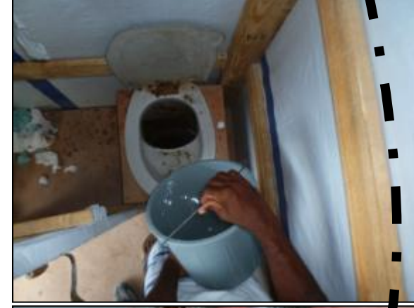
PHOTO T17 Unclogging urine bowl in UD seat
