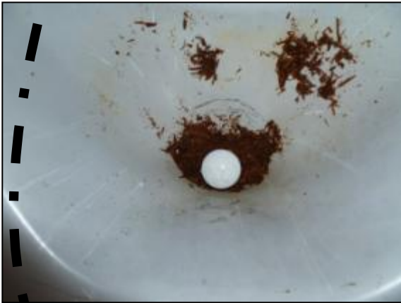
PHOTO T17 Unclogging urine bowl in UD seat
