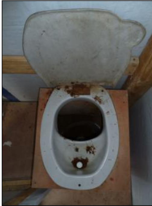
PHOTO T17 Unclogging urine bowl in UD seat
