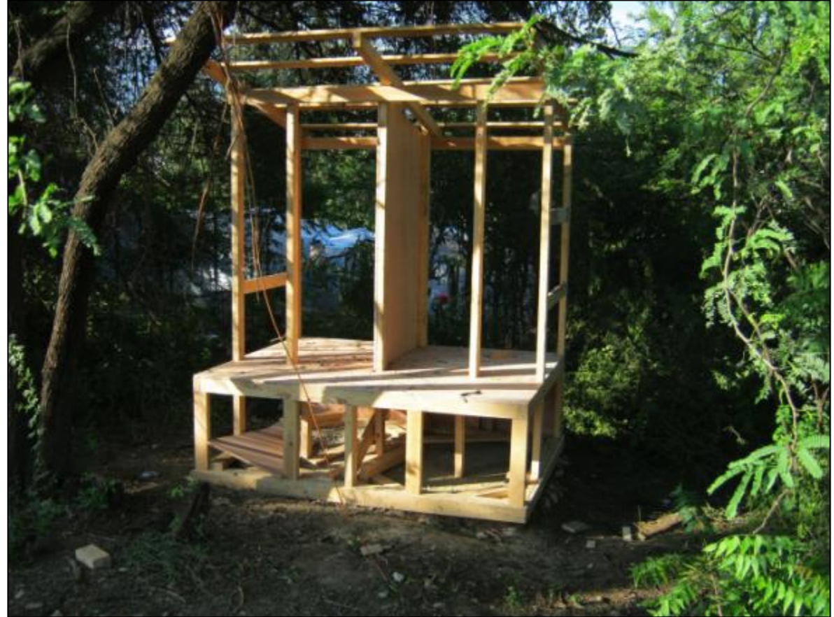
PHOTO T10: Wooden Structure
