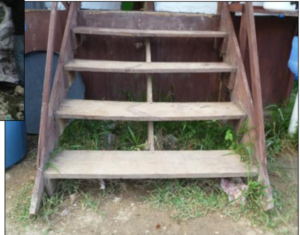
PHOTO T8: Stairs with central support
