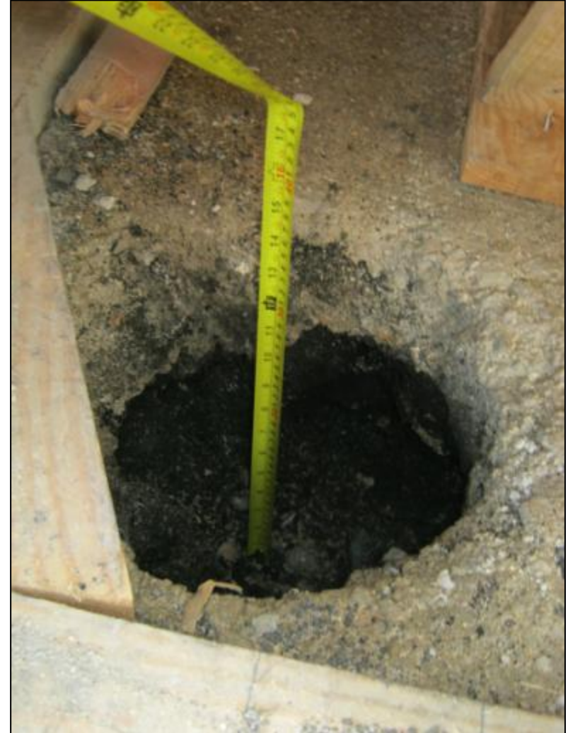
PHOTO T4: Urine Soakaway pit
