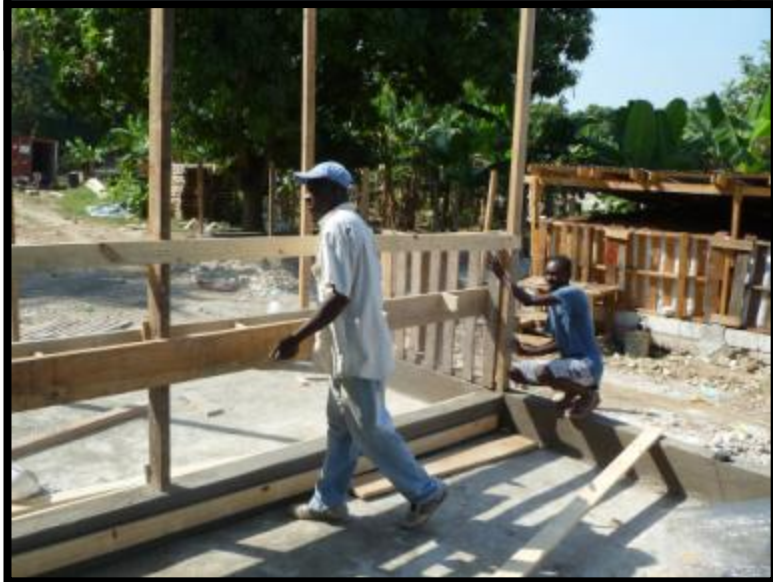
Photo K112: Interior walls construction.
