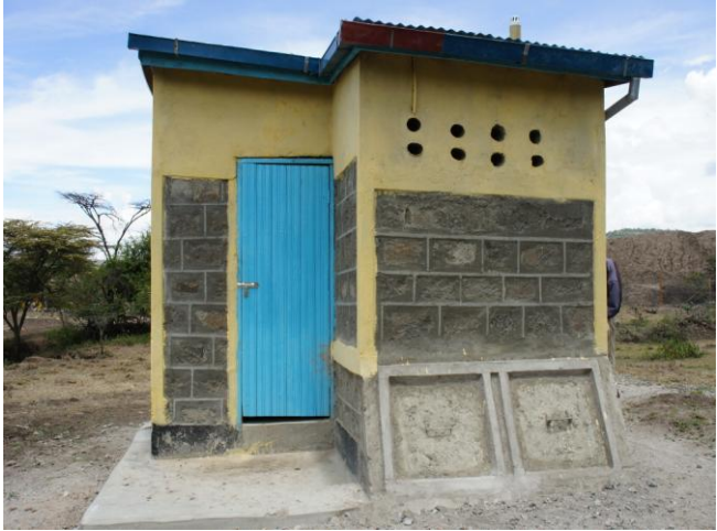
Ecosan, showing washing area and (sealed) access to composting chambers
