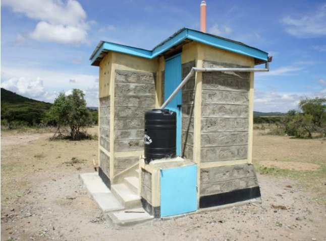
Male ecosan, with small rainwater harvester for hand washing
