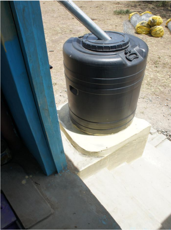
Male ecosan, with small rainwater harvester for hand washing
