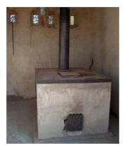
**Fig. 9:** Medical waste incinerator constructed on the Health Center's compound, 2004 (source: EcoSan Club)
