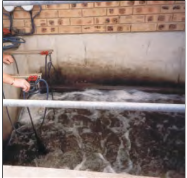
The operator cleans the sump and collects any debris. The debris is disposed of with the screenable material at the inlet (see page 8)
