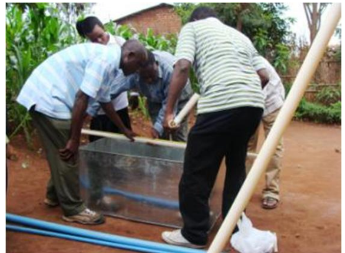
Fig. 6: Construction of the greywater treatment box (source: A. Ilberg, 2010)
