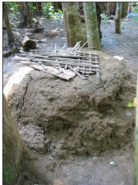
Pit latrine in flooding-prone area
