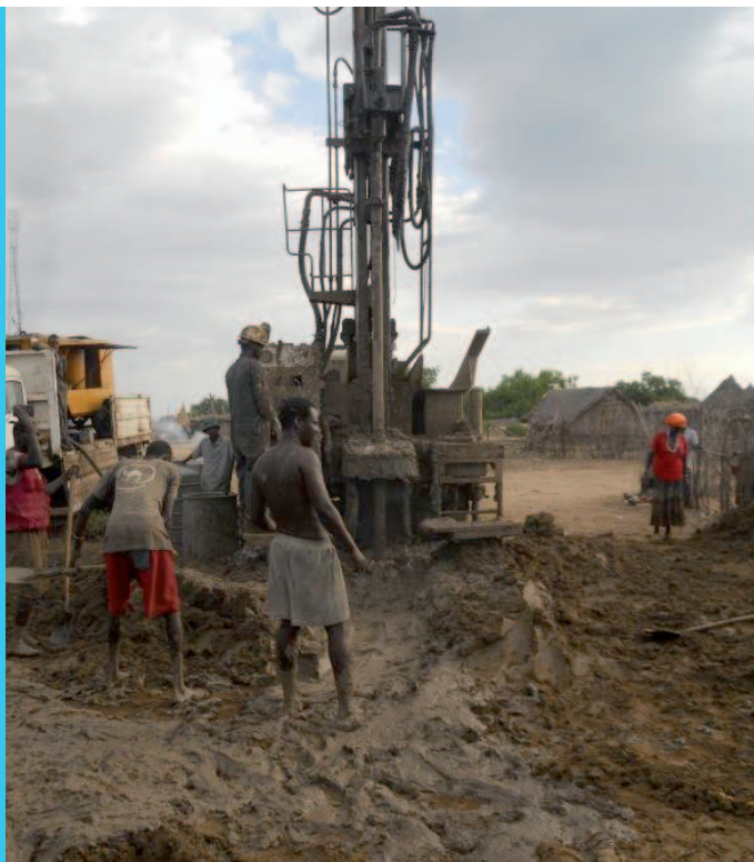
Figure 2. Borehole drilling, Ethiopia.
