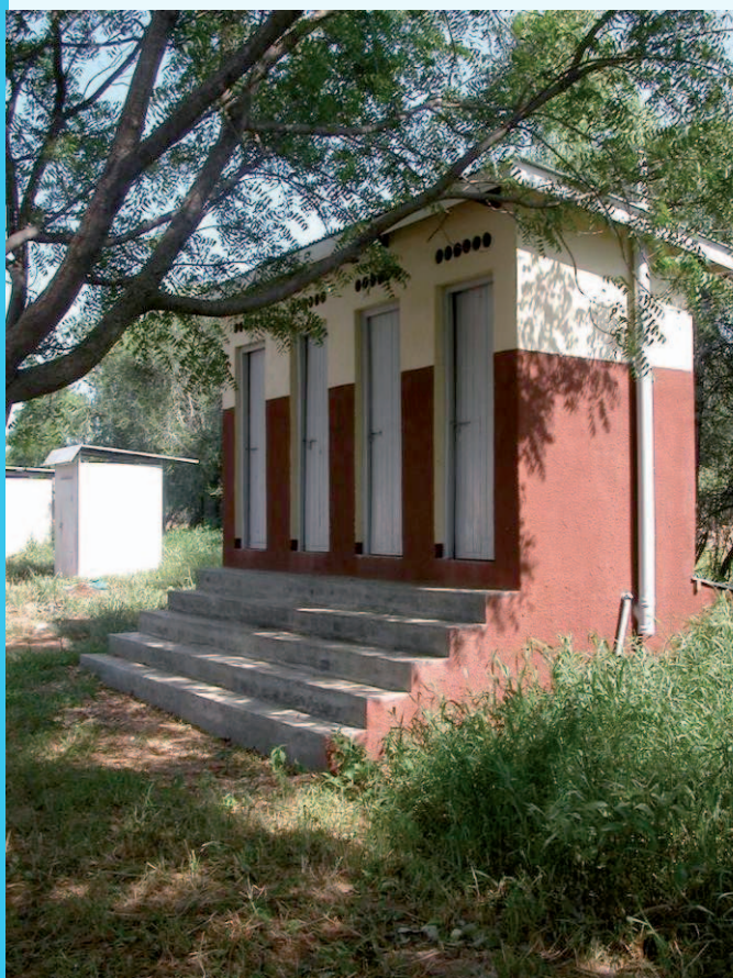
Figure 8. Composting toilets (rebuilt from pit latrines) at Kanawat Health Centre.
