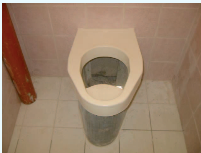
Figure 3. Toilet seat for a Urine-Diversion Dehydration Toilet (UDDT).
