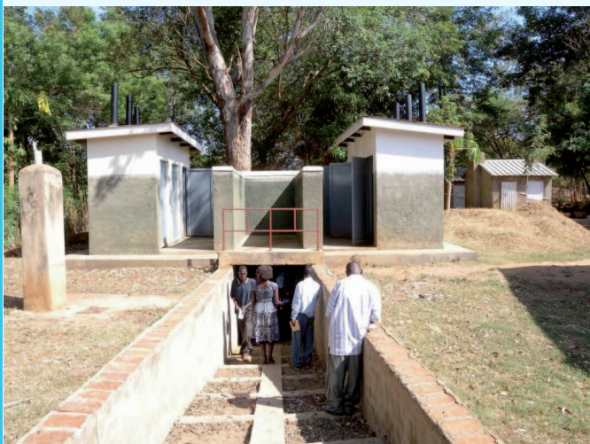
Figure 10. Toilet facilities at St. Joseph's Hospital.
