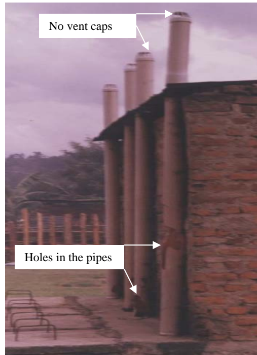
Figure 4.5a. A Solar dry-Toilet with a broken vent pipe Figure 4.5b. A Composting Toilet with broken PVC pipes
